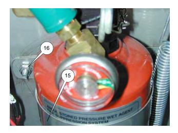
7. Disconnect the piping (17) from the fire extinguisher.
