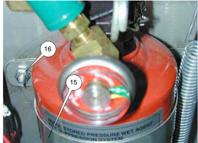
7. Disconnect the piping (17) from the fire extinguisher.
