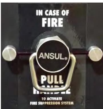
**IMPORTANT:** The manual pull handle is to be pulled ONLY IN CASE OF FIRE in the fryer (use when the automatic system has failed).
