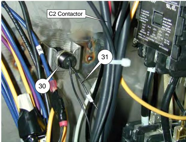
The Grease Filter Switch (30) is mounted to the interior wall in front of the C2 Contactor.
