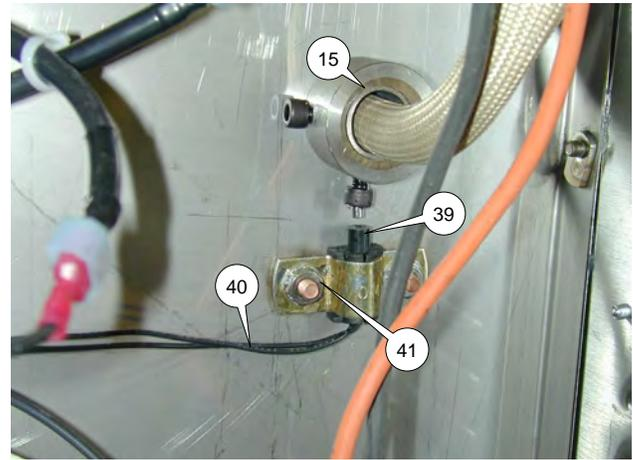
The Element Up Switch (39) is located in the control compartment on the interior wall below the Element Pivot Shaft (15).
